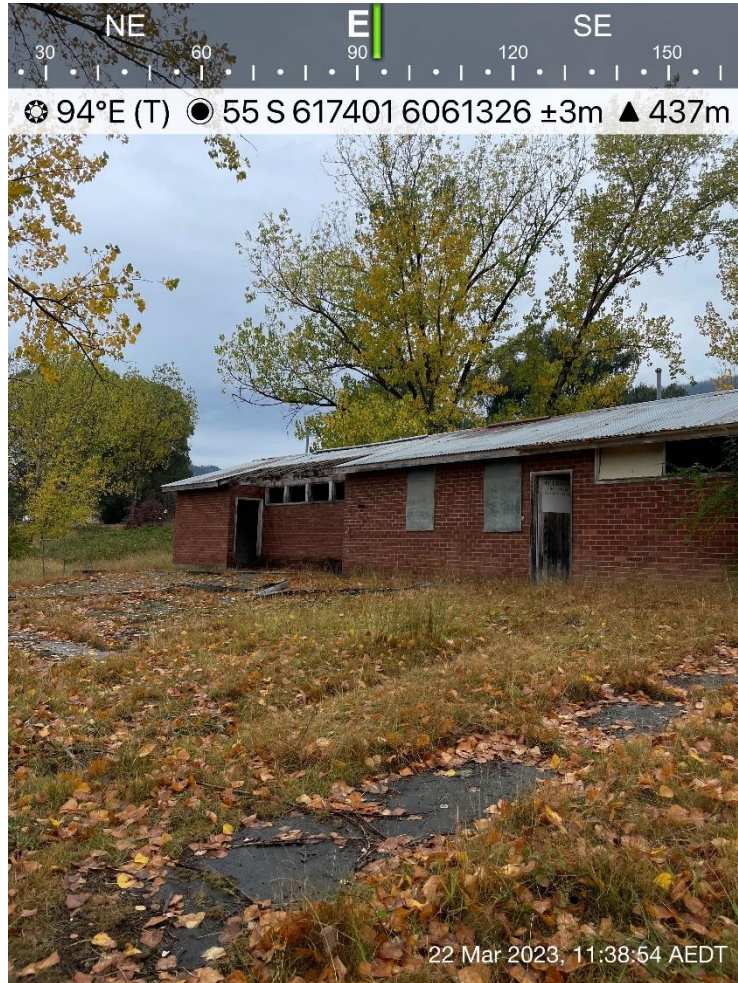
Photo 25: General view of an existing structure (former Talbingo Fire-Squad Training Area) located in the eastern section of the site.
