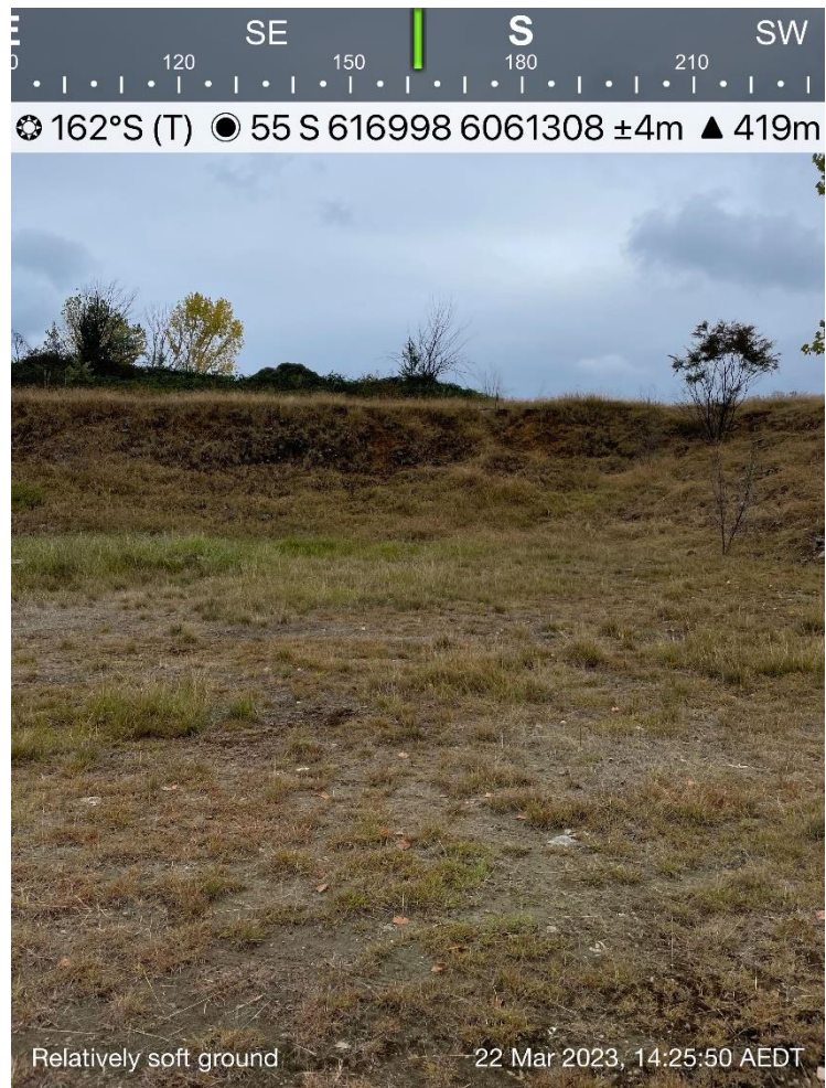
Photo 17: General view of the relatively soft ground located in the southern corner of the bottom of the up to ~ 6 m high embankment.
