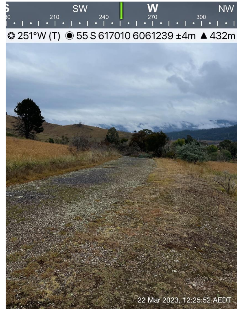
Photo 2: General view of an asphaltic sealed road off Wilkinson Street
