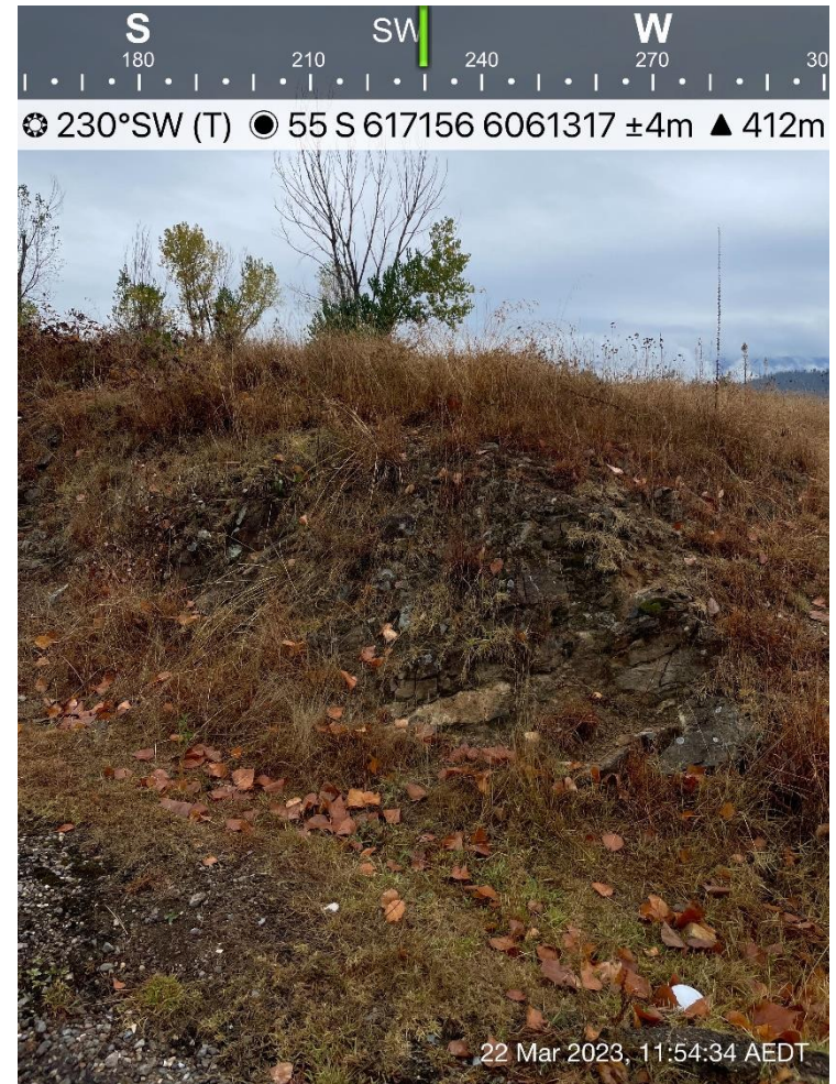
Photo 22: General view of weathered rock exposed in the embankment at the northern portion of the site.
