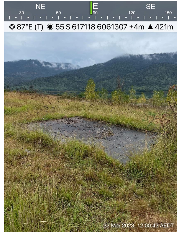
Photo 10: General view of a concrete slab located at the northern section of the site on top of the ~6 m high embankment.
